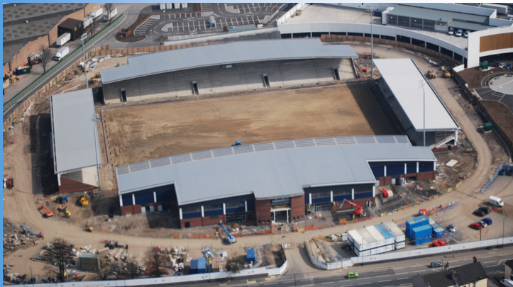
Latest progress photo
