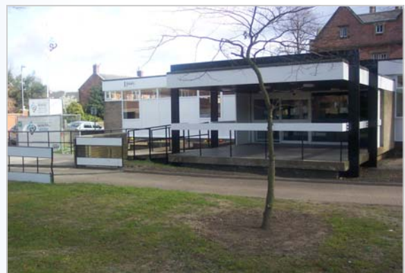
Completed Morpeth Library following flood damage
