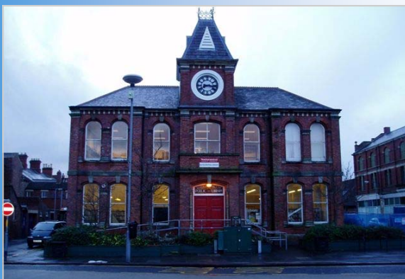
Completed roof works at Blyth Library
